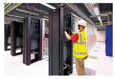
By routing cool air from the raised floor directly through the servers, equipment racks and cabinets, Skanska targets only the areas that require cooling. Our technique also minimizes unused white space that wastes cool air and forces the CRAC units to work harder without benefiting the temperature of the data center. A variety of other steps help enhance energy efficiency.
